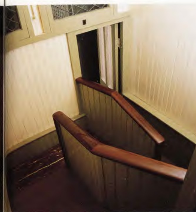
The switchback staircase has seven turns
