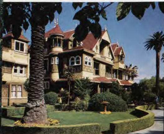
The façade of Llandra Villa, above, San Jose, California. Right: A wax effigy of widow Sarah Winchester, who acted as her own architect. Far right: The many skylights were thought to have been built to dispel the bad spirits' shadows.
