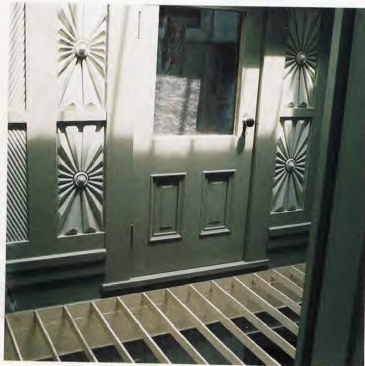
Slats added to prevent a two-story plunge
